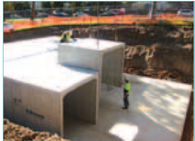
Concrete storage tank under construction using Humes precast components
