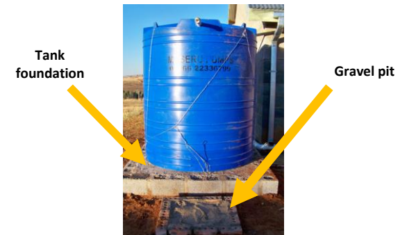
Figure 6. Picture of completed system in Motloheloh
