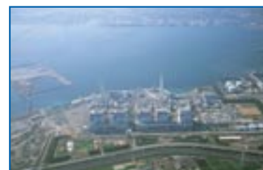
▲Hekinan Thermal Power Station
