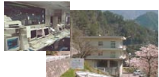
▲Oigawa Dam Control Center
