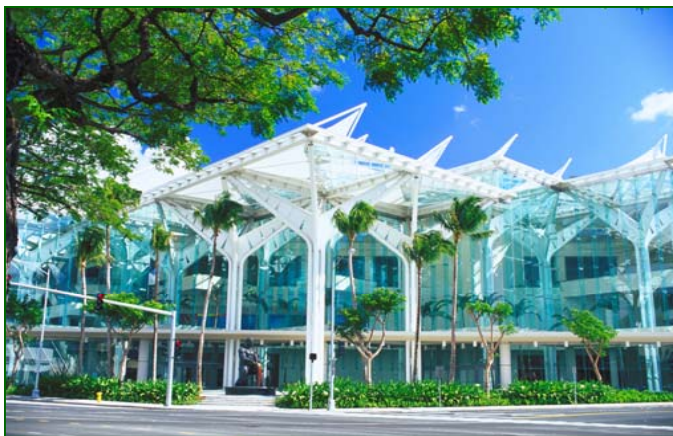
The Hawaii Convention Center is a state-of-the-art facility with 350,000 square feet of meeting and exhibit space. The Hawaii Tourism Authority oversees the planning and marketing of tourism in Hawaii.
