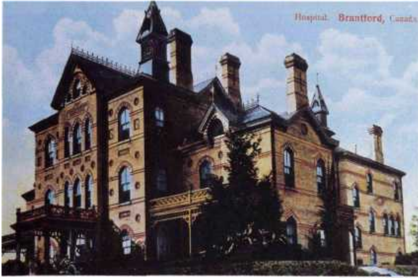
John Stratford Hospital, forerunner to the Brantford General Hospital, as it was in 1908.
