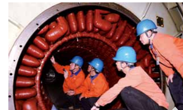
Inspection of equipment
