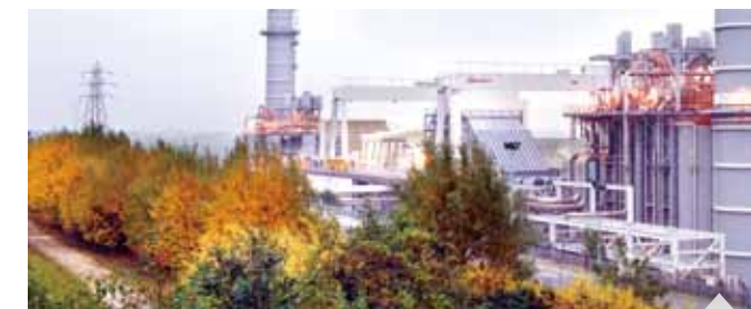
Britain Rocksavage Power Plant
