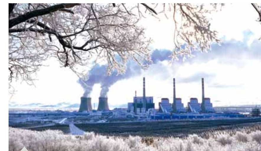
Yimin Power Plant
