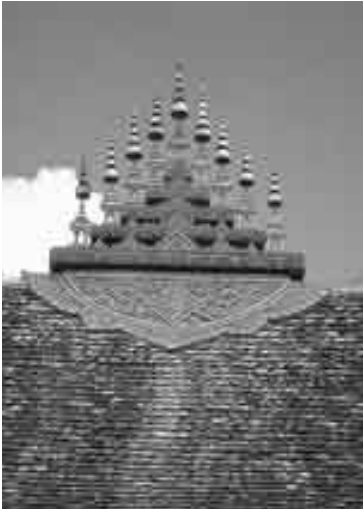
▲ The dok so fa , a particular feature of Laotian sim , is located at the centre of the sim roof ridge.
