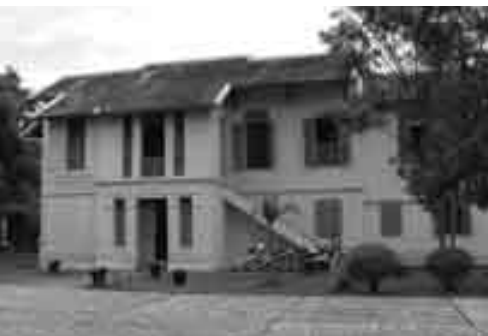
▲ Formerly the French colonial Customs House, this building was restored and converted for use as the offices of La Maison du Patrimoine. (Photo: Sirisak Chaiyasook)
