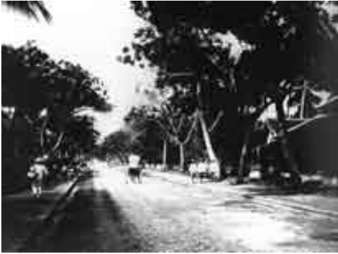
▲ In the 1920s tourism had just begun in Luang Prabang. This photo shows the main street at that time. (Photo: Reproduced with courtesy of the publishers of “Treasures of Luang Prabang”: the Institute of Cultural Research - Lao PDR, and the Cultural Association of the Silk Routes)
