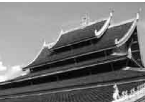
▲ This temple roof was recently restored using imported Thai roof tiles. While the end result may be attractive to some, the authentic Laotian heritage value of the site has been lost. (Photo: Rik Ponne)
