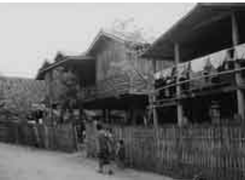
▲ Traditional Lao houses are built with bamboo, thatch and wood, with the quality of the materials depending on the wealth of the owner. They are usually free-standing structures, rectangular in plan and elevated on piles.
