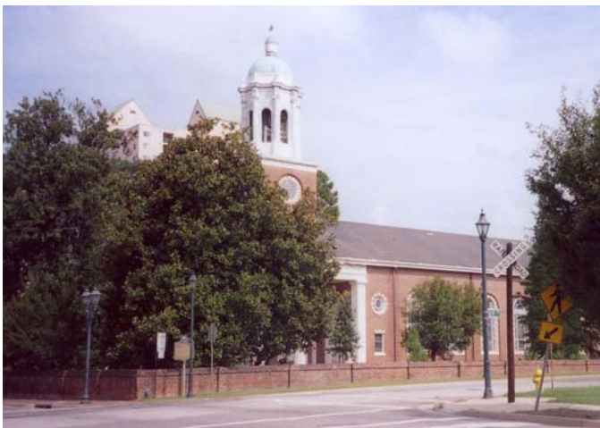
Saint Paul's Episcopal Church was first established in 1749 and was erected adjacent to the Fort Augusta. In 1758 the Parish of Saint Paul was created for administration of Augusta and the surrounding countryside. The current 1811 building, pictured above, is the third church to occupy this site. 11
