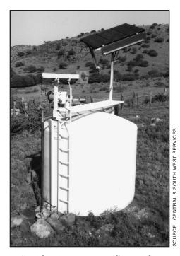
Using the sun to water livestock This PV system powers a small pump jack sitting atop the water storage tank. During sunny weather, when cattle are most thirsty, PV watering systems perform at their peak.
