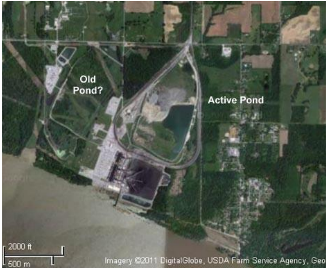
Joppa Steam Plant Ash Ponds, Joppa, IL.
