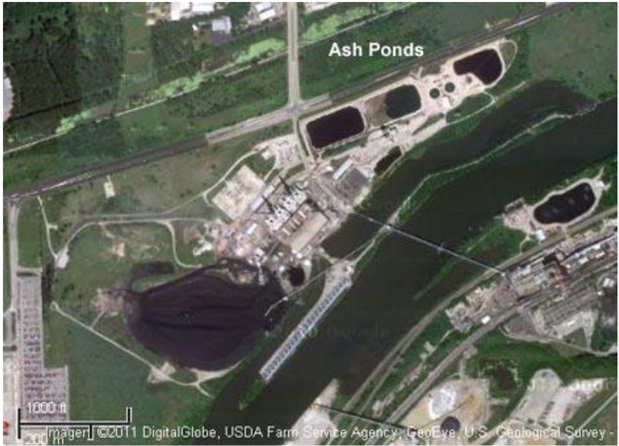
Joliet 29 Generating Station Ash Ponds, Joliet, IL.
