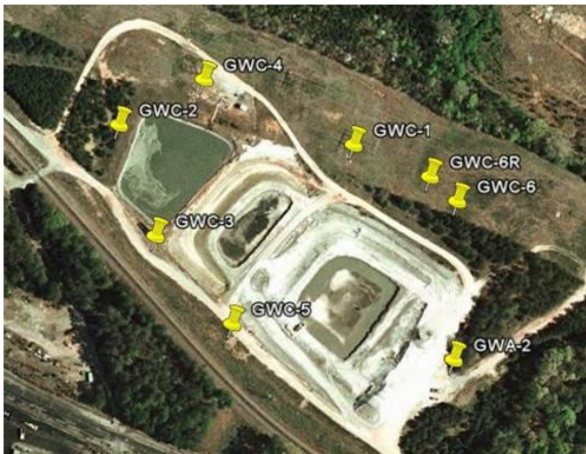
Yates Generating Plant FGD Landfill and Monitoring Wells.
