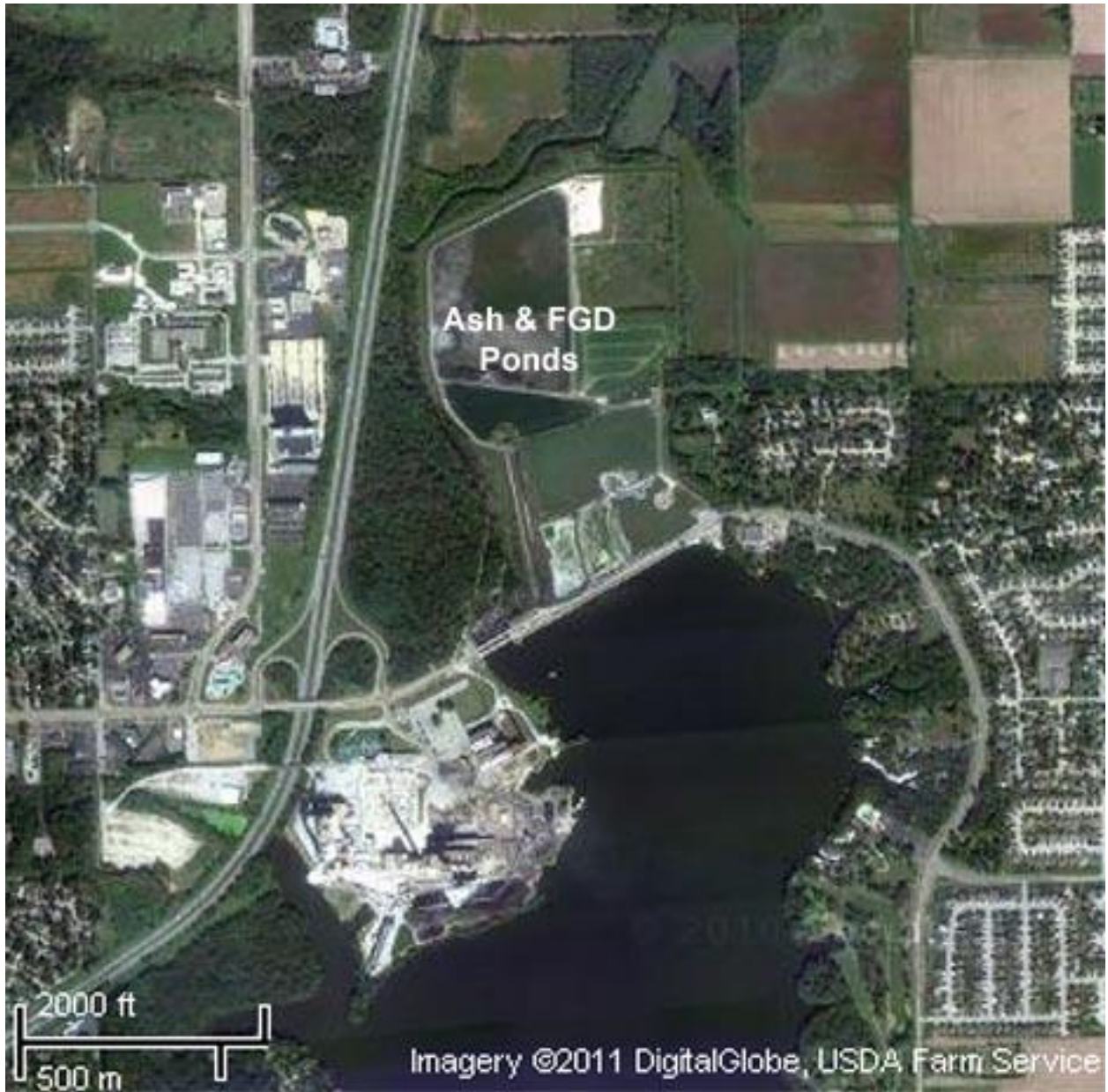
Dallman Station Ash and FGD Ponds, Springfield, IL.
