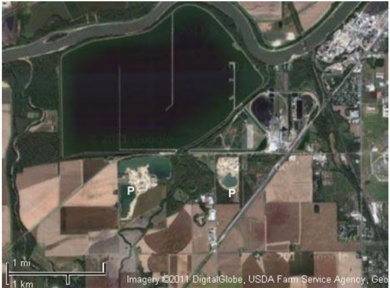
Powerton Generating Station Ash Ponds (P), Pekin IL.
