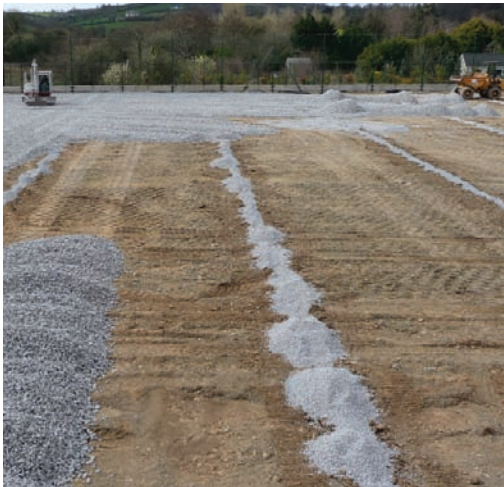
Construction of unbound base
