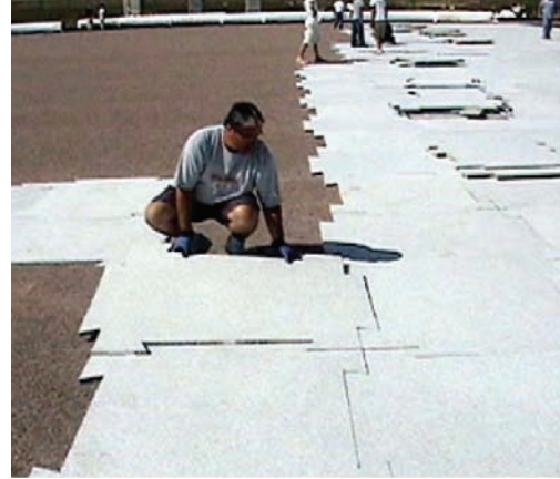
Preformed panel pad being laid on unbound base
