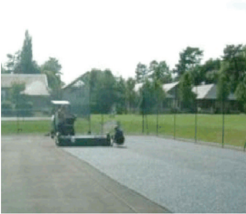
Insitu rubber pad being laid on macadam base.
