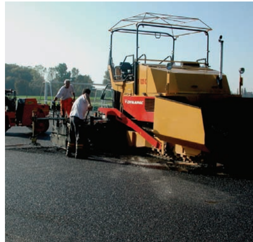
Construction of bound (macadam) base
