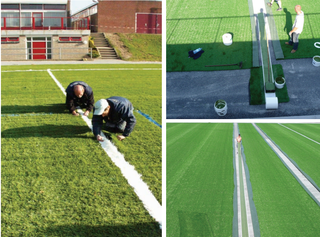
Carpet installation process.
