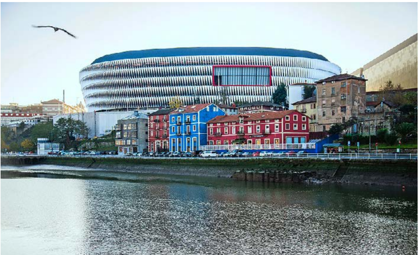
Bilbao's new pride and joy: Some sections of the San Mames stadium are still under construction.
