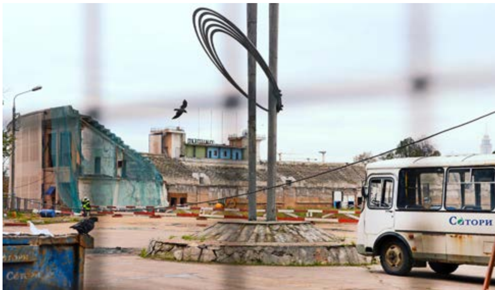
Under construction: Russian football must overhaul its infrastructure for the 2018 World Cup (picture: Dynamo Stadium).
