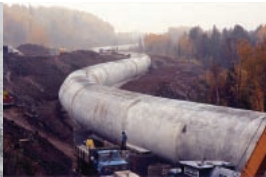
1997 construction of single new aqueduct
