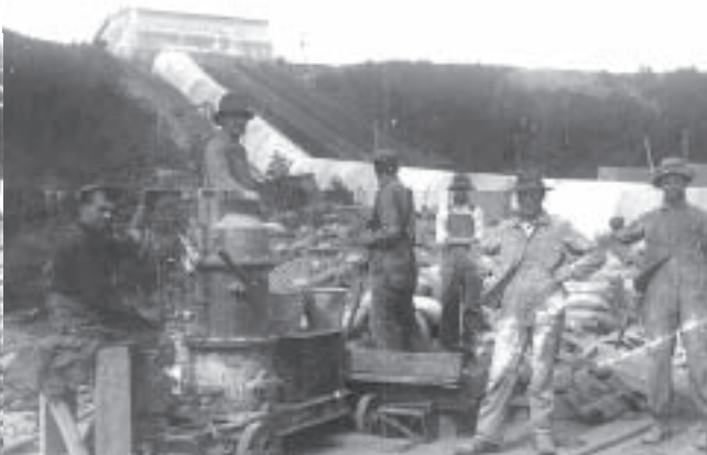
Construction - Penstock and surge chamber in the background.
