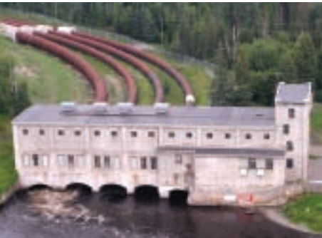
Kakabeka Falls Generating Station
