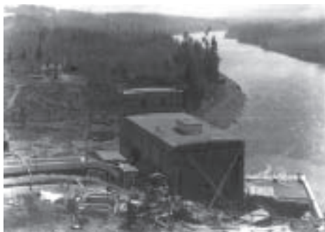
Overview of construction site. Superintendent's house in the background, circa 1906.
