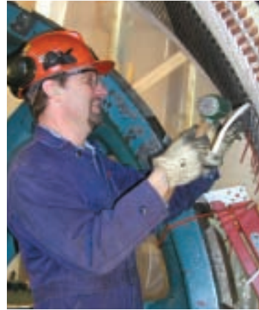
Working on the generator rewind
