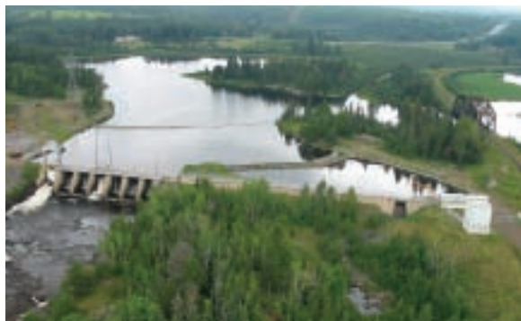
Main dam and intake structure
