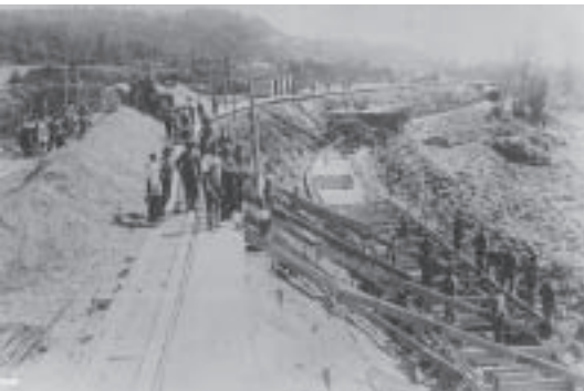
Construction of the original third aqueduct in 1914
