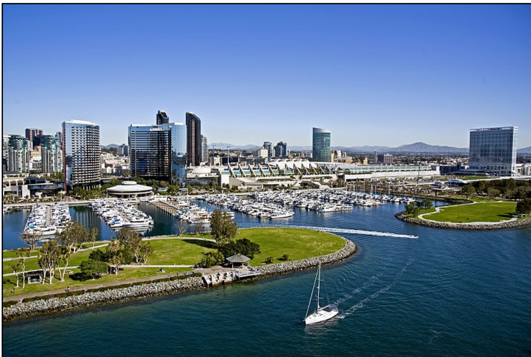
Figure 1: Overview of the SDCC Facility
