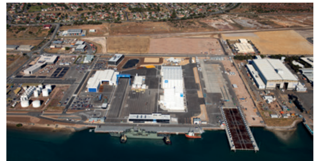
FIGURE 8.1: ASC SOUTH (LEFT), COMMON USER FACILITY (MIDDLE) AND ASC NORTH (RIGHT), ADELAIDE
