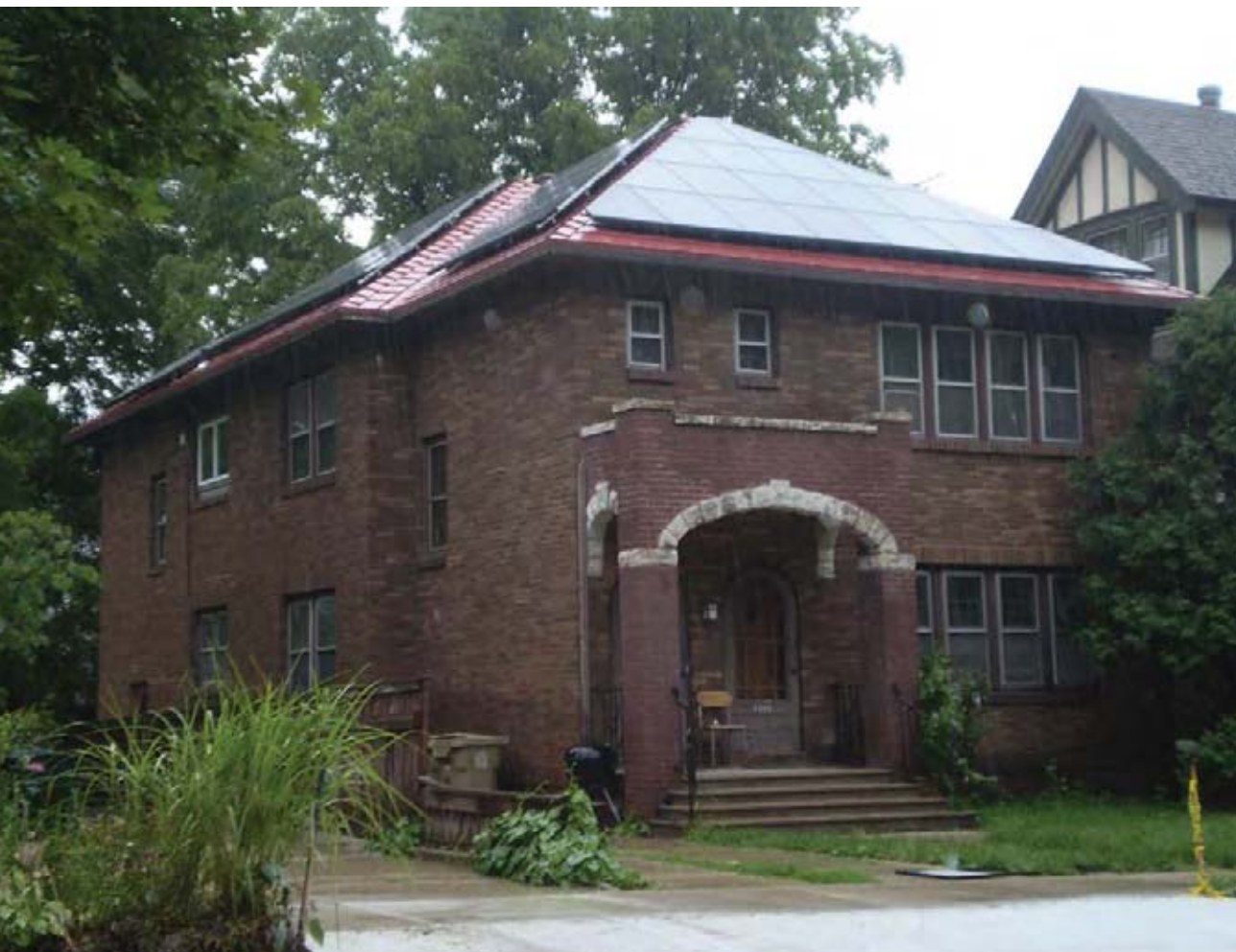
The owners of this home installed a triangular shaped PV array system so as not to compromise the design integrity of this historical home. (Vipin Gupta/PIX17930)
