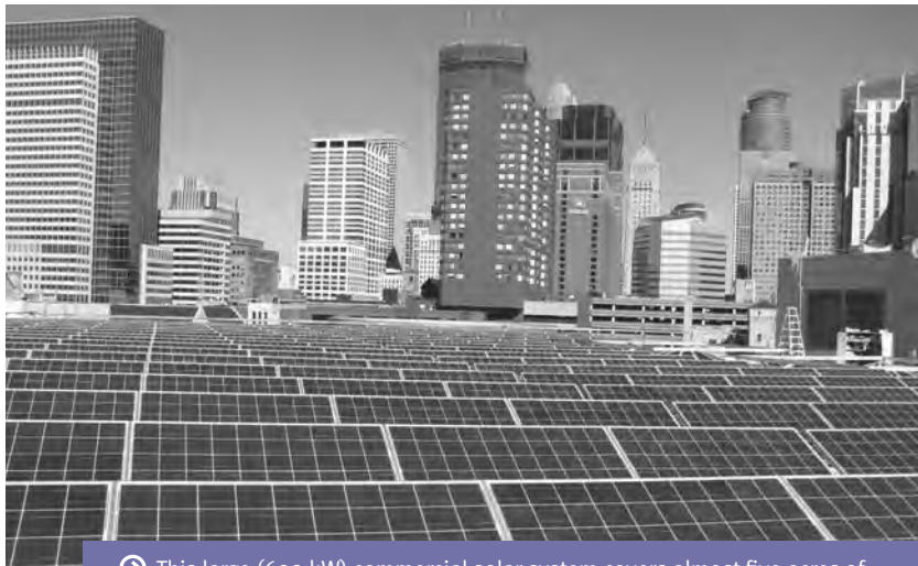
➡ This large (600 kW) commercial solar system covers almost five acres of rooftop as an accessory use at the Minneapolis Convention Center.
