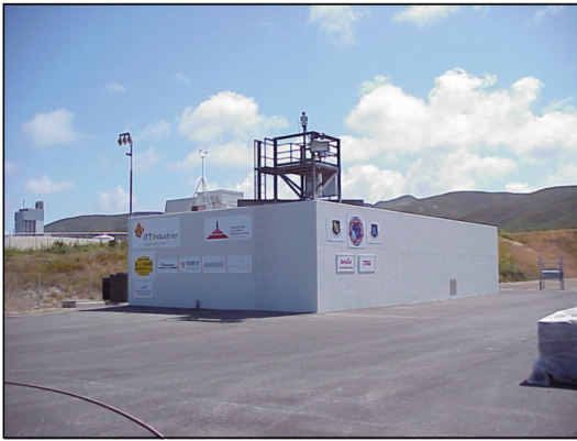
Figure 4-1: Support Equipment Building
