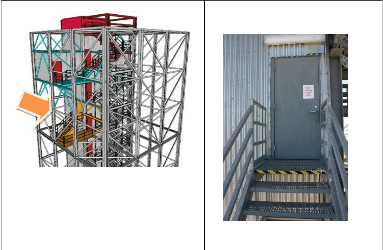
Figure 3-11: New Level 3 Access
