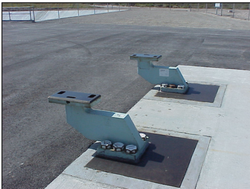
Figure 5-1: T/E Pylons Installed at the Spaceport
