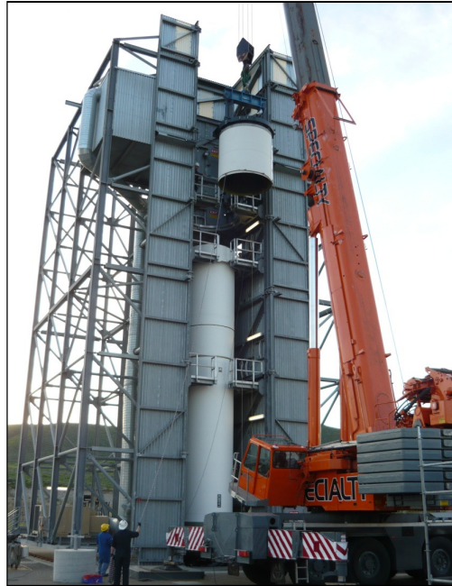
Figure 5-5: Minotaur IV Stage 3 Stacking Operation Using a Portable Crane
