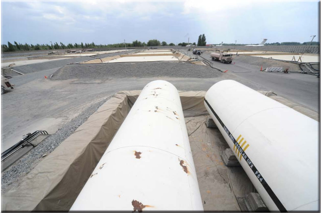
Fuel bag farm at Manas Transit Center Photo Credit: Air Force Staff Sgt. Nathan Bevier
