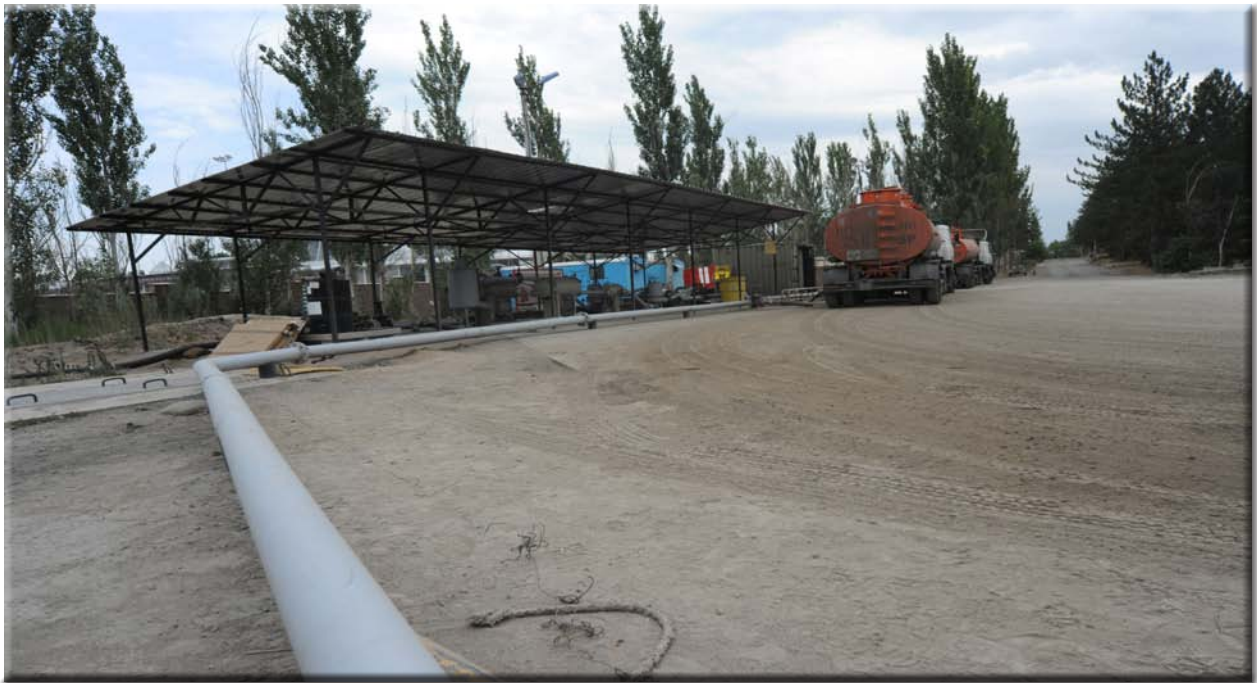
Offloading header outside Manas Transit Center fuel bag farm Photo Credit: Air Force Staff Sgt. Nathan Bevier
