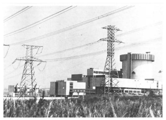
Heat is extracted from the 1000-MW WWER nuclear power plant at Novo-Voronezh in the USSR to supply nearby industrial consumers with hot water and steam.
