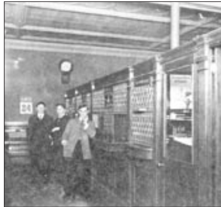
The interior of the bank showing the decorative, and protective, cast-iron tellers' cages.
