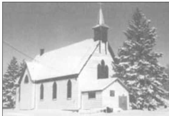
Extensive renovations were made to the original 1876 church in the 1950s. A kitchen and parish hall were added in the 1960s.
