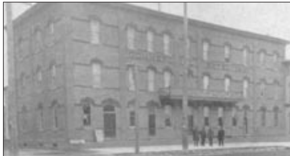
The Commercial Hotel as pictured in A Souvenir of Seaforth published in 1900. You can clearly see the horizontal bands linking the window arches and sills of each storey. Pilasters mark off four sections vertically across the facade. Note that there are four separate entrances. The hotel proprietor at the time was George E. Henderson.
