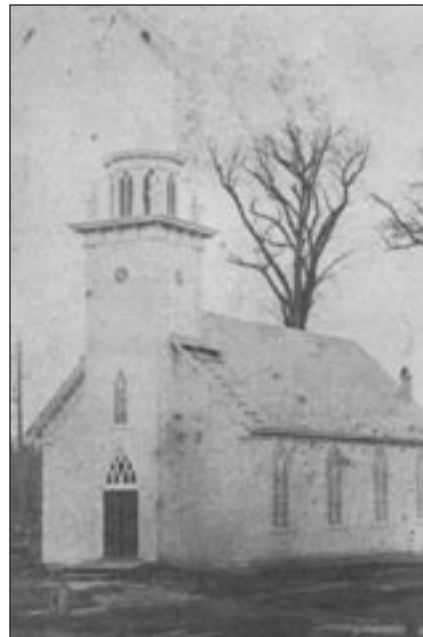
Building the Church in 1863.
