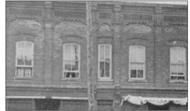
A – This block shows superb craftsmanship in the frieze brickwork.
