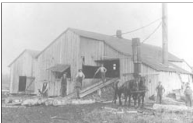
Querengesser Sawmill – the team hauled logs up the ramp and a “dolly” took the logs endways, placing them beside the saw carriage; logs were rolled onto the carriage by a canter using a cant hook. Lumber came off at the other end where it was piled by tailers.
