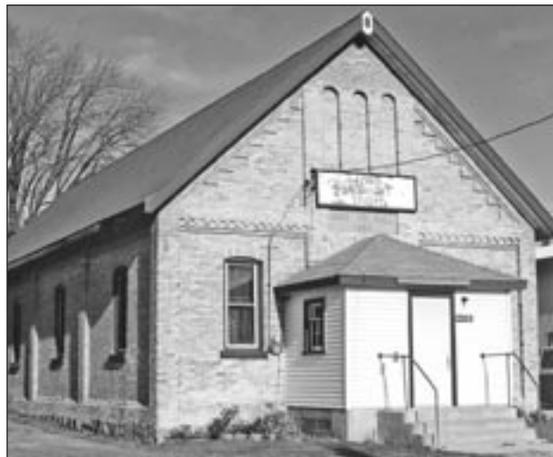
The date stone reads: Grey Tp. Hall 1892. Note the raised decorative brickwork of the gable end and the pilasters marking the corners and bays.
