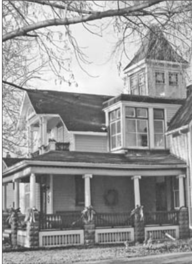
Lavoie House has many features of the Queen Anne Revival style of late Victorian architecture.
