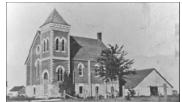
Knox Presbyterian Church was built in 1911, replacing the original church. It is now a residence.
