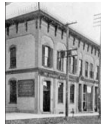
The Canadian Bank of Commerce in the Dominion Block at 94 Main St S.
