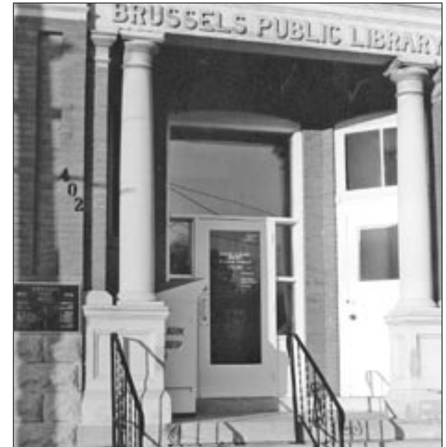
The classically columned portico of Brussels Public Library.
