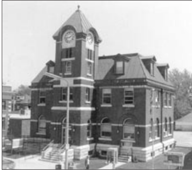
Note the rusticated stone foundation and the use of the white stone in the banding.
