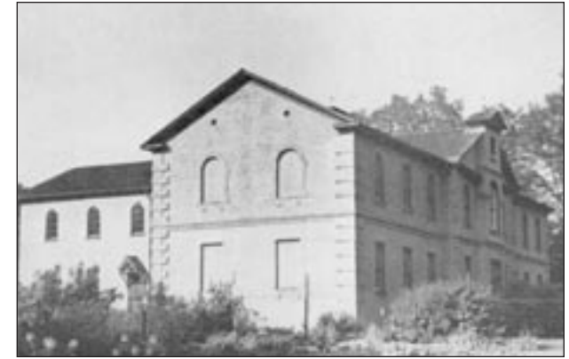
A view of the south side with the addition made in 1872. Note the central front door.
