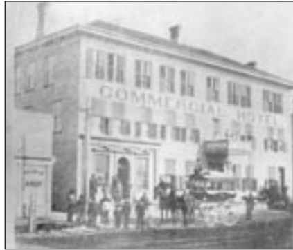
The original Commercial Hotel built by Thomas Knox in 1866. The photo was taken some time before 1893 when the barbershop at the left of the picture was torn down to make way for the town hall.
