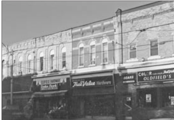
Note the decorative brickwork in red and white.
