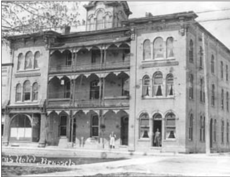
The Queen's Hotel was a centrepiece on the main street. Belden described its "two projecting wings ... a handsome piazza of equal height with the main building, the centre topped by a lofty and highly ornamental rectangular tower." It was torn down in 1986.
