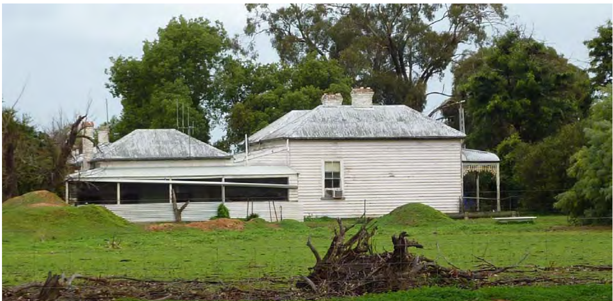
West elevation, viewed from Oxleys Road. The c. 1864 brick dwelling is pictured left. The larger weatherboard structure was relocated from the nearby New Nil Desperandum Mine in c. 1916.
