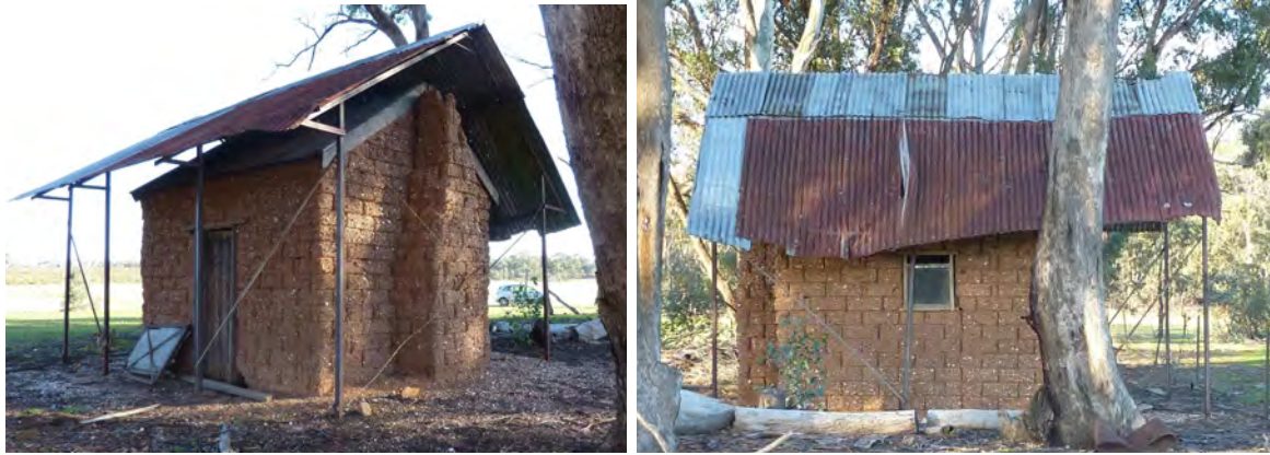
Left: Sleeping quarters, looking north-east. Right: West wall. Note damage to protective enclosure caused by a falling branch.
