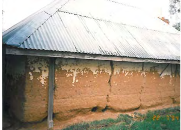
Left: The former farmhouse. Right: Mud brick structure, possibly the 'cooling chamber' of the former dairy. (Source: Both pictures are dated 22 July 1994 and supplied by the City of Greater Bendigo.)
