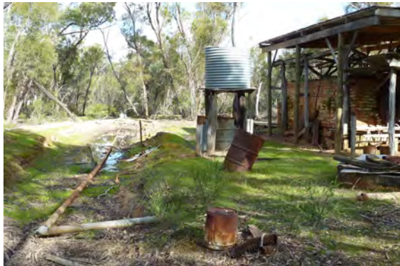
Left: Brick and stone-lined condensing dam. Right: Base of former stack at rear of boiler.
