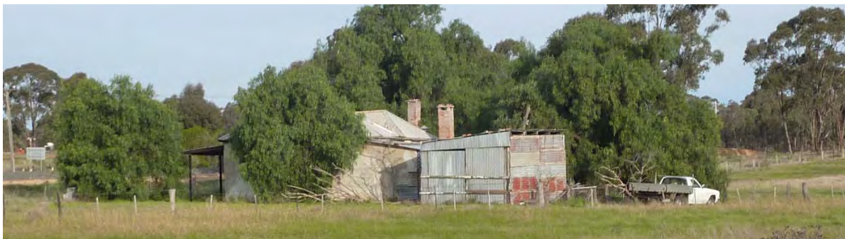
Rear of the Engi farmhouse property, viewed from Sebastian Road to the north.
