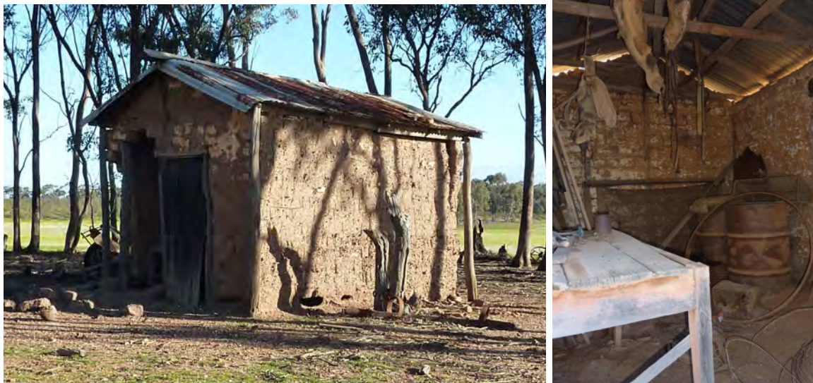
Left: Dairy, south and east walls, note fallen mud bricks to the entrance. Right: Dairy interior.
