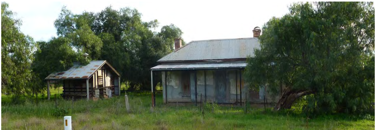
Front (east) elevation of the Engi farmhouse, with outbuilding to the south (left).
