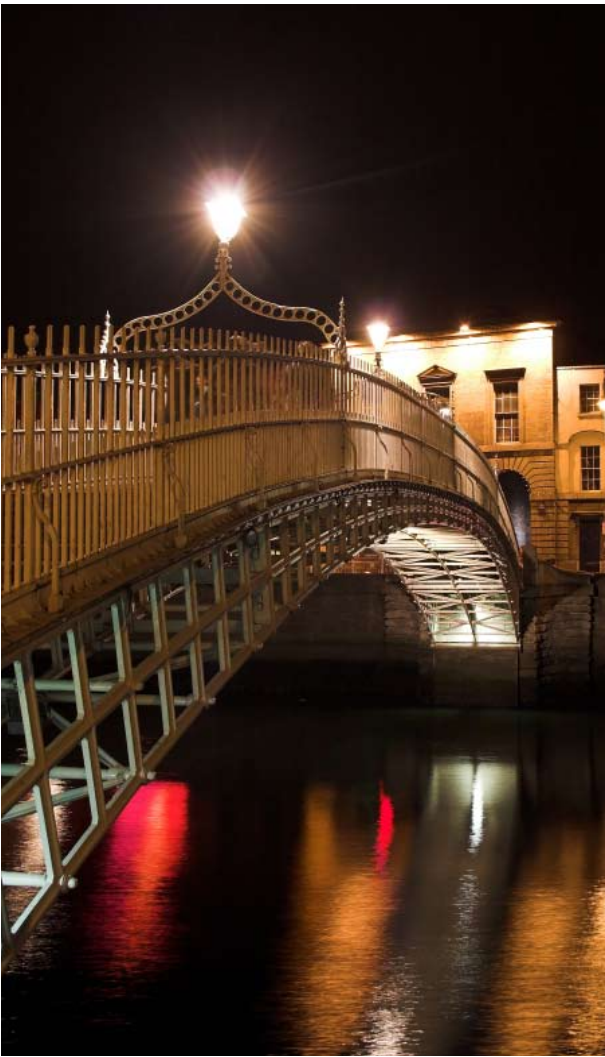
Figure 120: View of the Ha'penny Bridge, Dublin.
