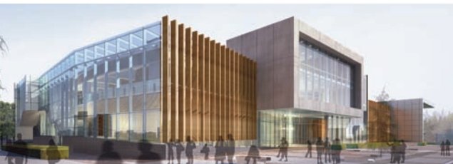
The new LEED Gold-certified Centre for Engineering Innovation at the University of Windsor will address broad challenges facing the automotive sector. Photo: supplied
