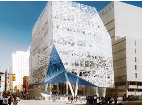
Ryerson University's impressive Student Learning Centre is expected to be complete by winter 2014. Photo: supplied
