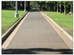
SECONDARY & MINOR AVENUES Secondary Avenue Width: 4 metres Minor Avenue Width: 3 metres Paving: Asphalt Kerb & Gutter: Pre-cast concrete units
