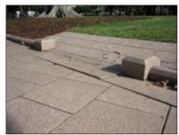
MAIN AVENUES Width: 1.8 metres Paving: Granite unit paver Border: Pre-cast concrete units
