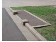
SECONDARY AVENUES Width: 1.8 metres Paving: Asphalt Border: Pre-cast concrete units
