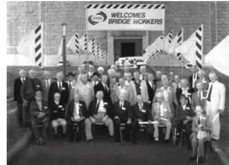
Bridge Workers in 1987 RTA Photographic Library Collection
