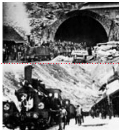
Construction of the Gotthard tunnel.
