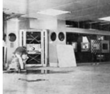
Construction of Union Bank agency, Zurich main station, 1970.
