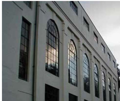
Bonnington Power Station, Lanarkshire
