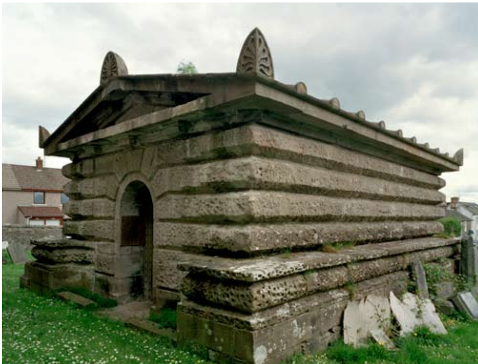
Lynedoch Mausoleum, Methven, Perthshire Crown Copyright: RCAHMS
