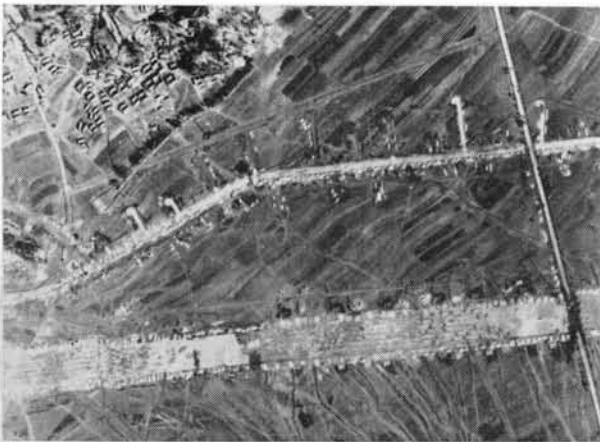
Figure 42. Rear Area Storage.
