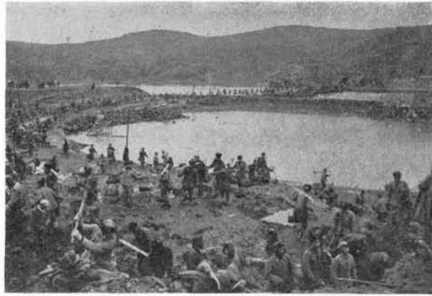
Figure 40. Troops Building a Reservoir.
