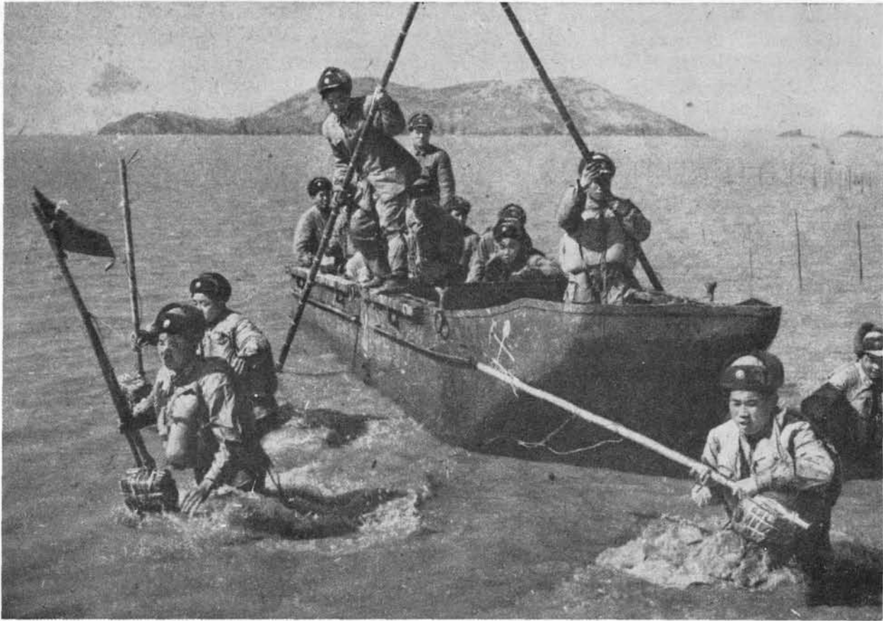
Figure 122. Steel Ponton Boat with Engineer Demolition Team.
