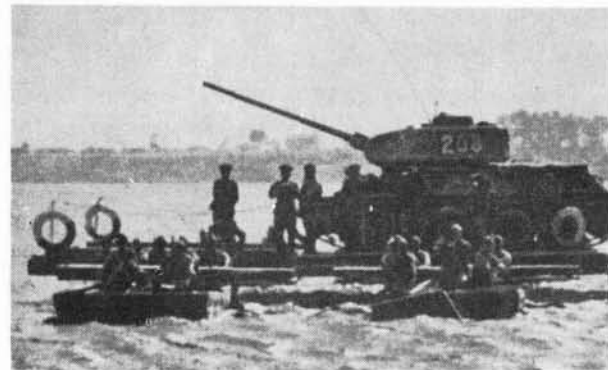
Figure 123. Ponton Ferry with T-34 (85) Medium Tank.
