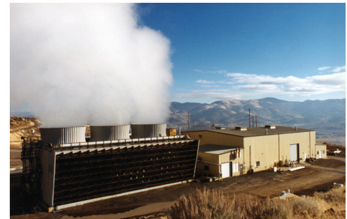
Steamboat Hills Geothermal Power Plant 31 Steamboat Springs, Nevada
