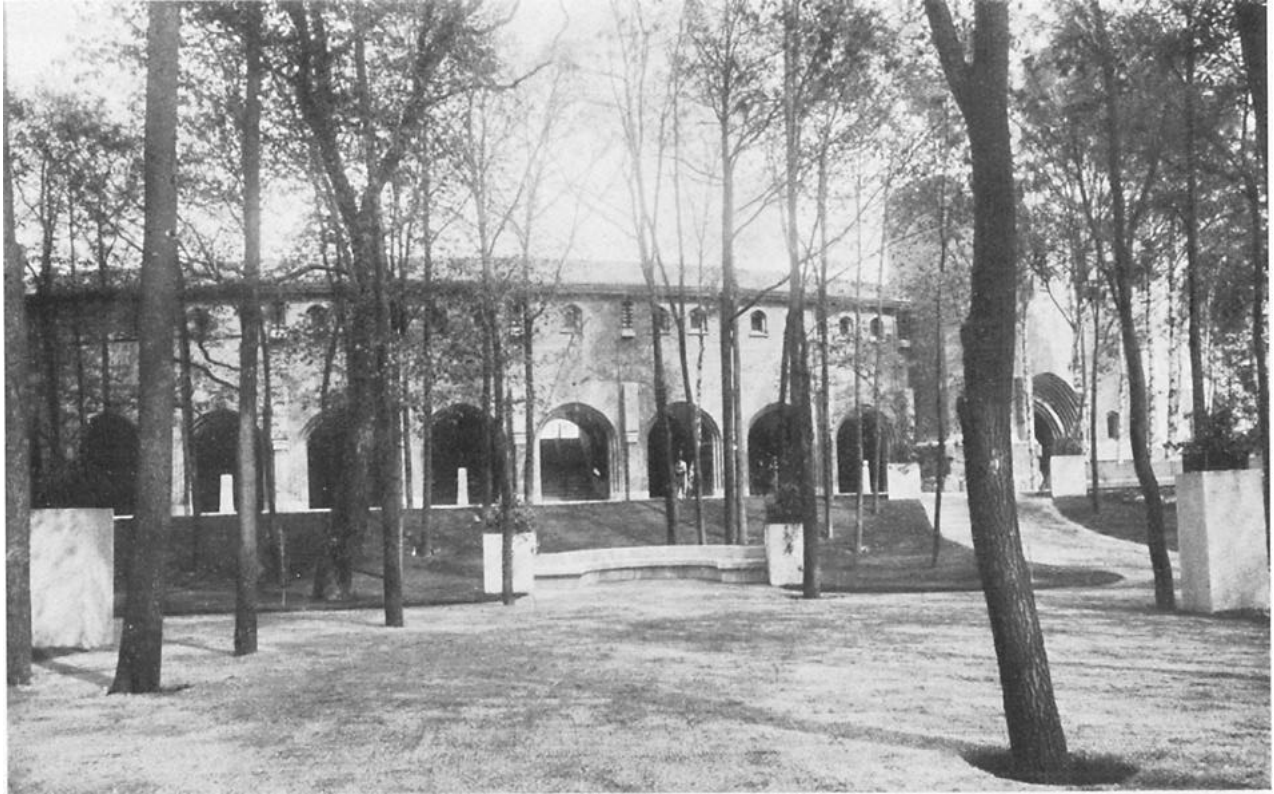
THE GARDENS AND SOUTH ARCADE OF THE STADIUM.
