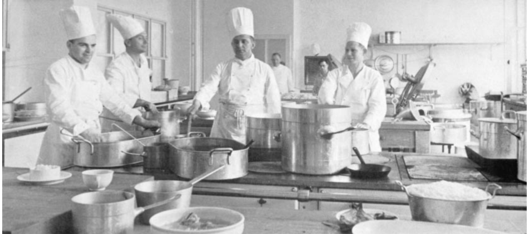
One of the large kitchens in the Household Building.
