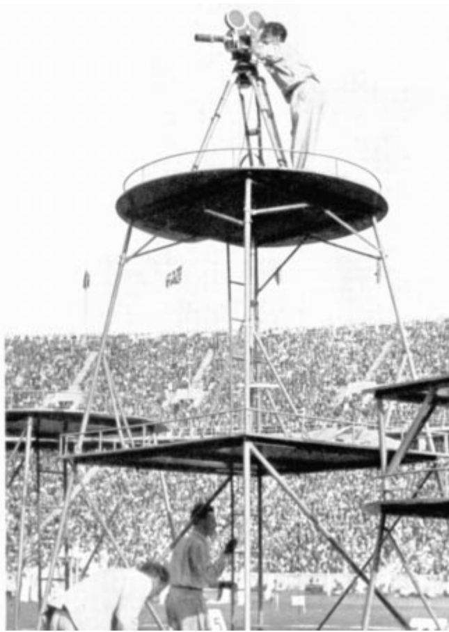
The tower erected in the arena of the Stadium.
