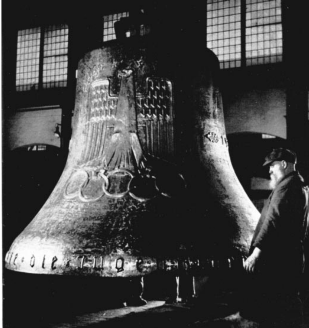
Cooling, polishing, chasing and tuning—and the Olympic Bell is completed.
