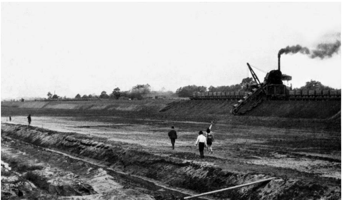
The Toda rowing course under construction.
