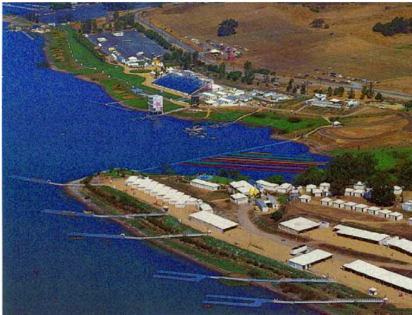
30 A natural lake is converted by the LAOOC for use as the site of canoeing and rowing. Note especially the unique temporary bridge for athletes between their area (foreground) and the spectator area (above right).
