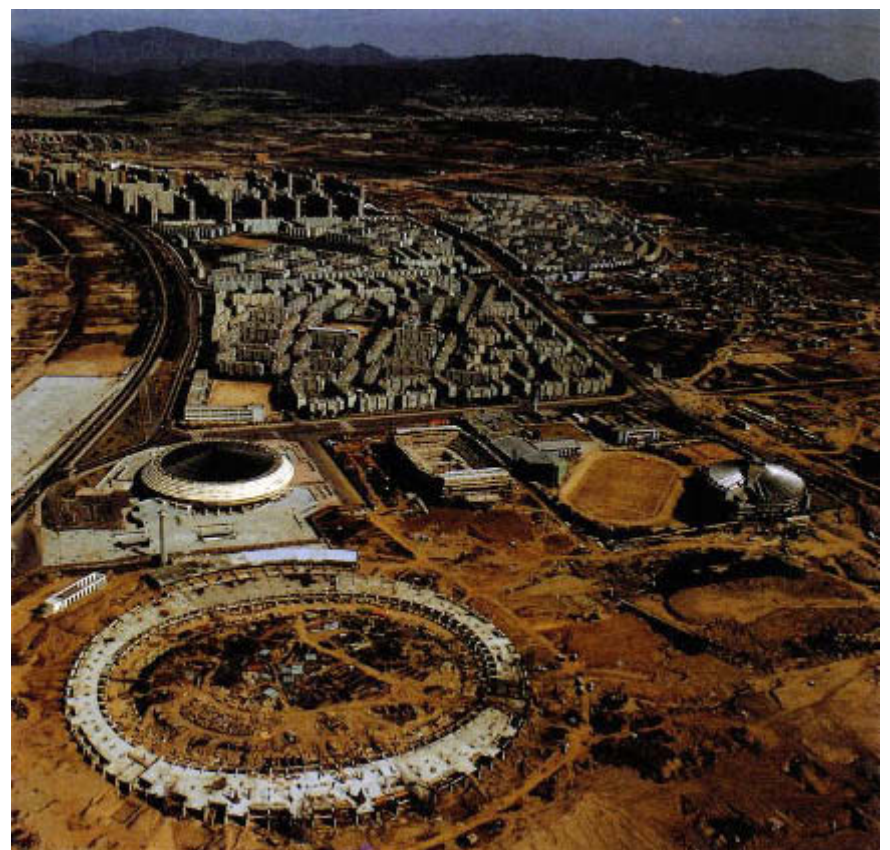
1. The Seoul Sports Complex during the early construction phase in 1979.
