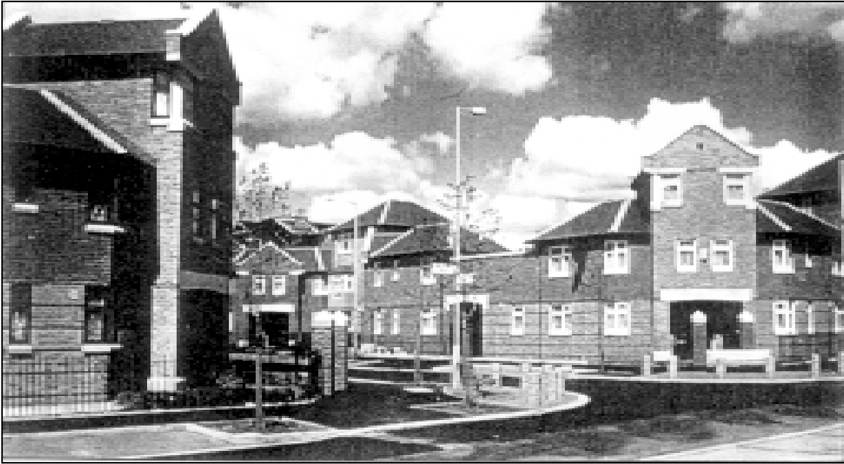
New housing in Chichester Road, Hulme, 1998
