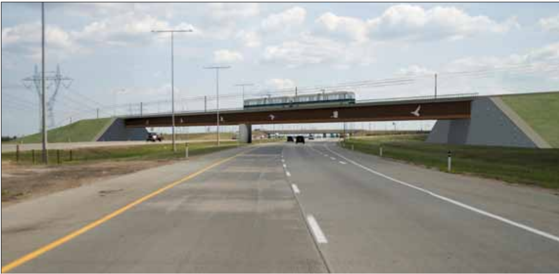
Anthony Henday Drive Bridge
