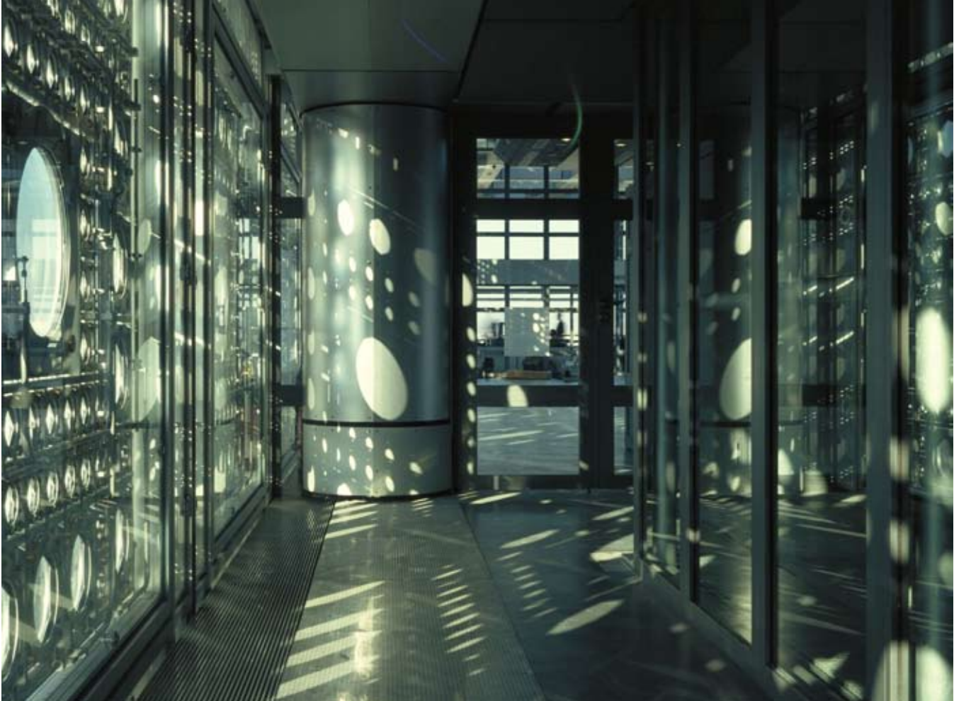
Institut du Monde Arabe (IMA or Arab World Institute) 1981-87 Paris, France above: exterior view of wall showing adjustable metal lenses below: interior view of the metal lenses Photos by Georges Fessy
