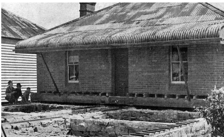
Figure 9 Moving House! The cottage after moving. DMR, Annual Report , 1950, opp p 12
