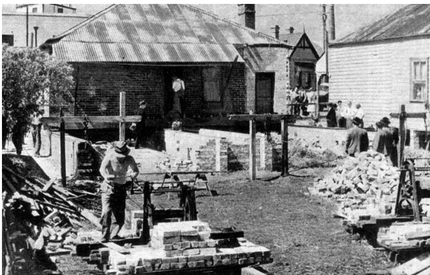
Figure 8 Moving House! A brick cottage affected by road widening was moved as an experiment by the DMR in 1950. This shows the cottage before moving. DMR, Annual Report , 1950, opp p 12
