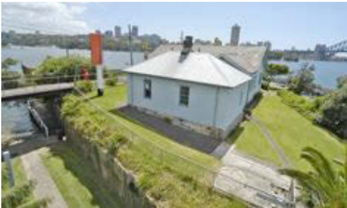
Figure 3.21 Overview of the precinct and the Cut.
