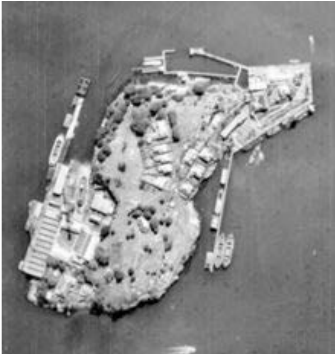
Figure 3.46 1968 aerial photograph of Goat Island, showing the maximum extent of wharves and buildings on the island
