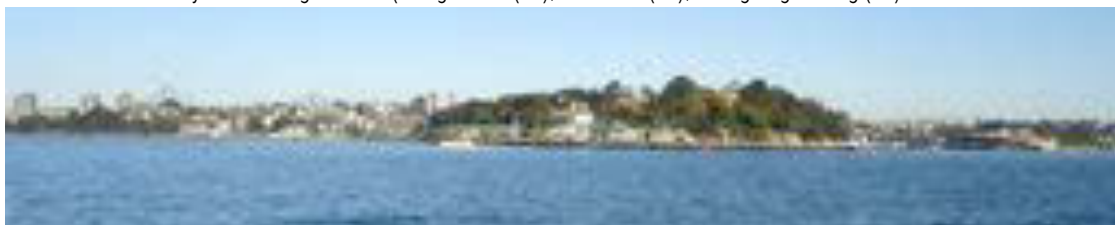
Figure 3.44 A more distant view of the island from the east. From this distance the northern built elements, particularly the Water Police Station (47) retain some visual dominance but the vegetated form dominates the view. The Harbour Master's Residence and adjacent cottages are virtually hidden by vegetation.
