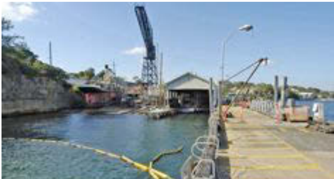
Figure 3.15 View of the shipyard precinct from wharf 4b
