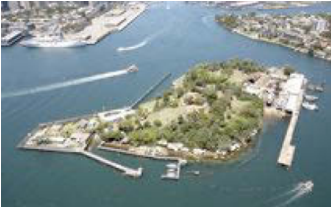
Fig 3.26 The north depot precinct is the narrow strip of land and the wharves that extend across the northern and eastern face of the island with the distinctive boat pens at the western edge of the area.
