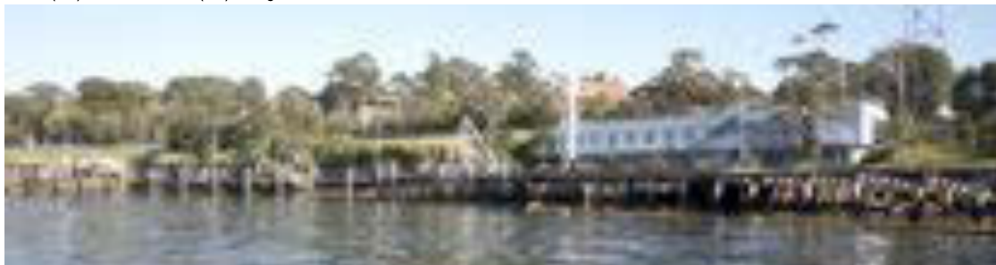
Figure 3.37 A close view from the north of the former eastern wharf (52) with the Wharf Mooring Floating Plant (51) visible on the far left. From this view position the wharves dominate the scene with the Port Emergency Services Building (45) being the most visually dominating element on the northern part of the island through its mass and light colouring, with the Harbour Master's Residence (39) visible behind.
