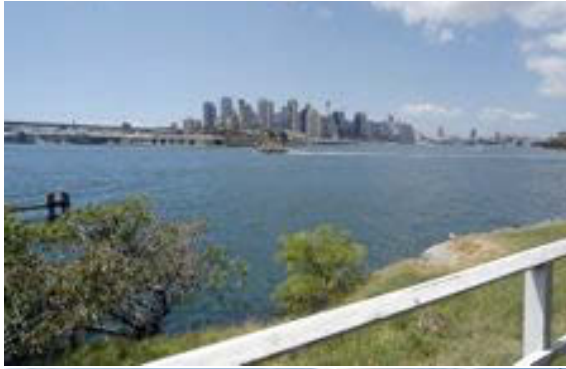
Figure 3.49 The view from the Magazine Walk (69) towards the city, taken from the Central Precinct and looking back towards Darling Harbour.
