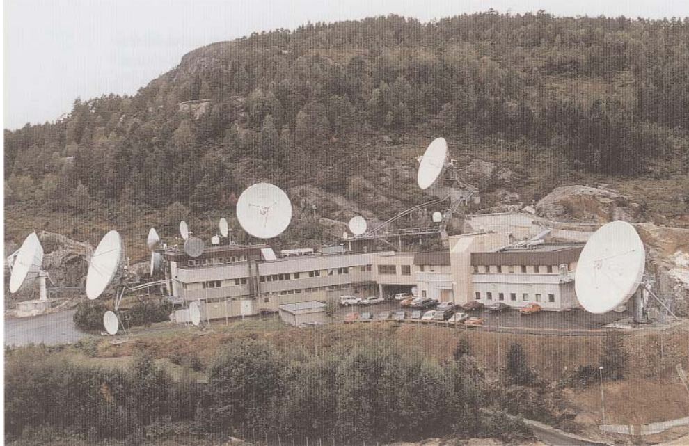
Eik earth station
