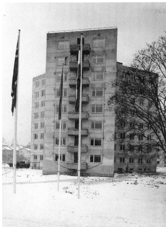
Figure 1 Ullevål accommodation facilities. The cables had to be laid on the outside of the walls and through the air vents to every room that was to be fitted with telephone
