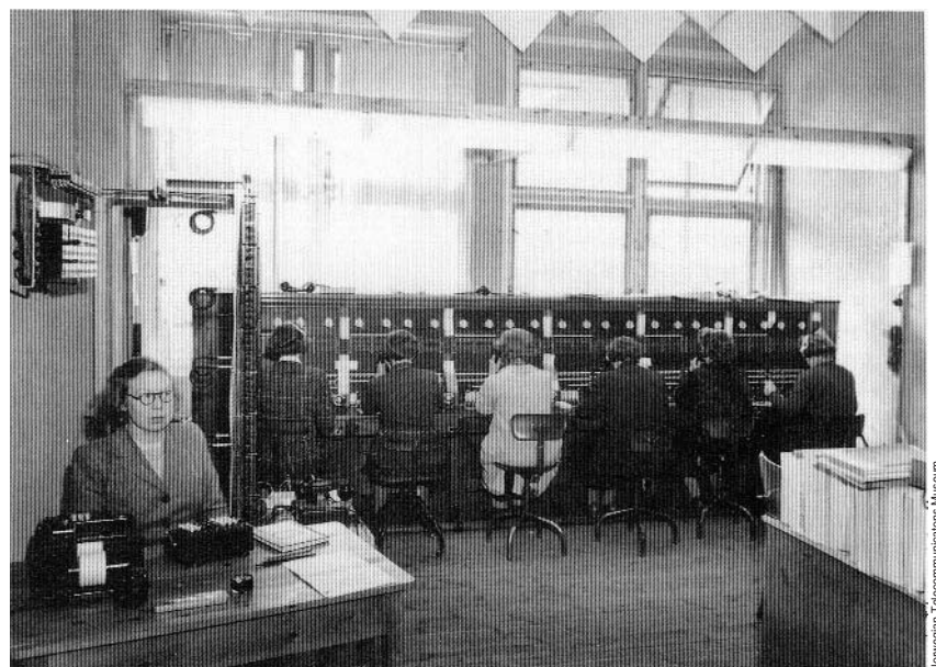
Figure 6 Long distance switchboard at Hotel Viking
