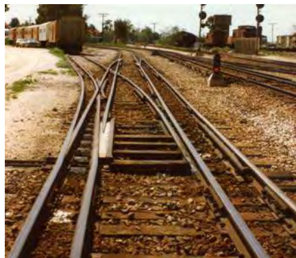
Turnout: (3 gauge) Main to (s.g+n.g) Branch. 2 moving blades and transition
