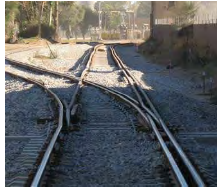
Turnout: (b.g+s.g) - Main and Branch. 3 moving blades
