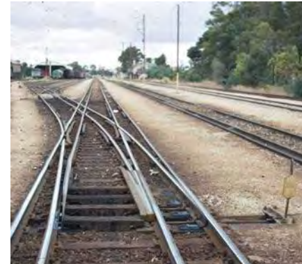
Turnout: (3 gauge) to (b.g+n.g) Branch. 2 moving blades
