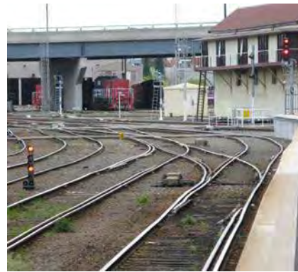
Transition: (b.g+s.g) Conventional transitions (both tracks)
