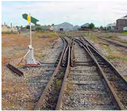
Turnout: (3 gauge) - Main and Branch. 4 moving blades
