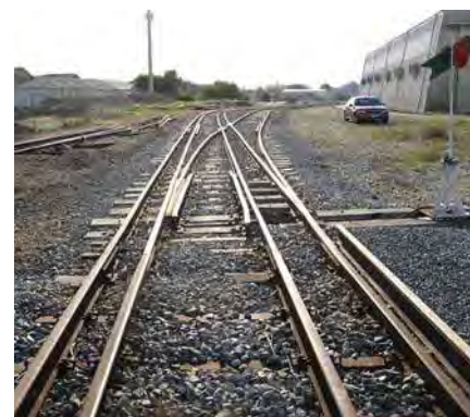
Turnout: (3 gauge) to b.g Branch. 1 moving blade
