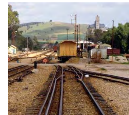
Transition: (3 gauge - common rail) to (3 gauge 'gauntlet')
