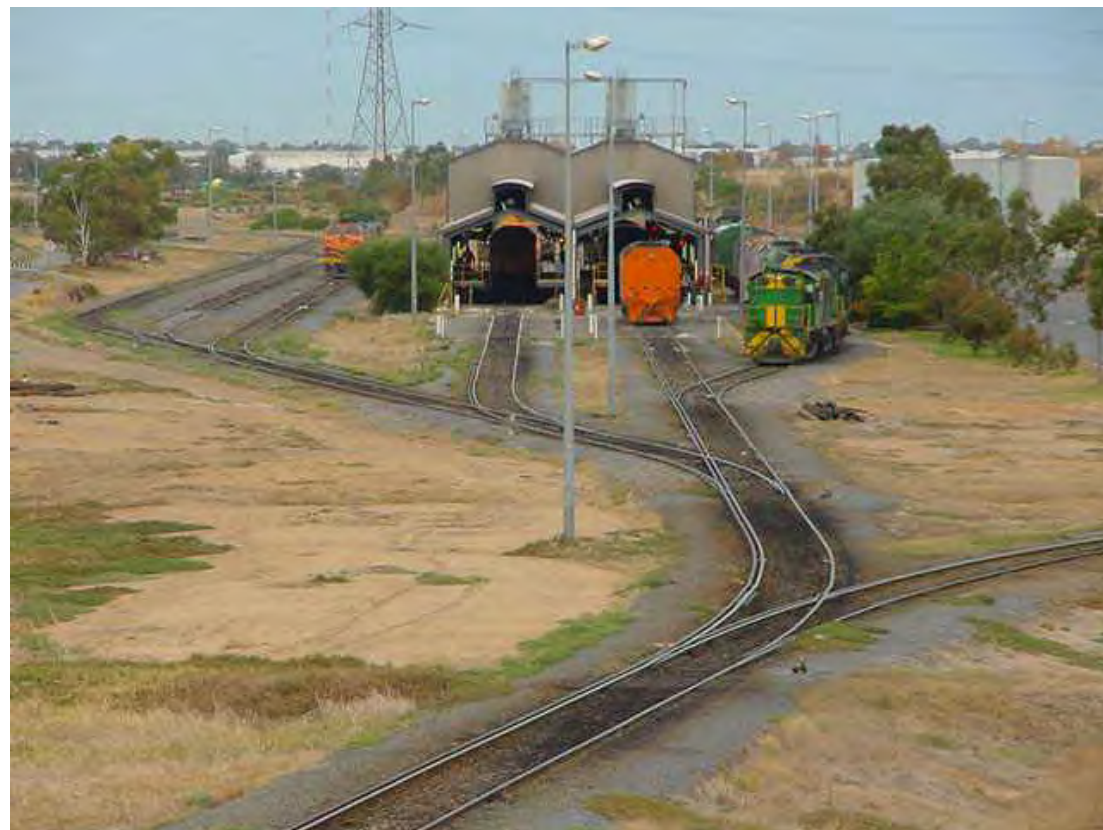
Dual Gauge at Dry Creek MPC
