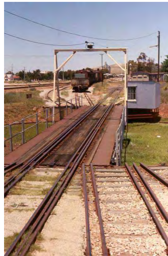
Triple gauge symmetrical (Note the standard gauge thin railhead)
