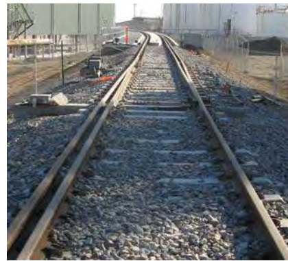
Transition: (b.g.+s.g.) Switched transition. 2 contra moving blades
