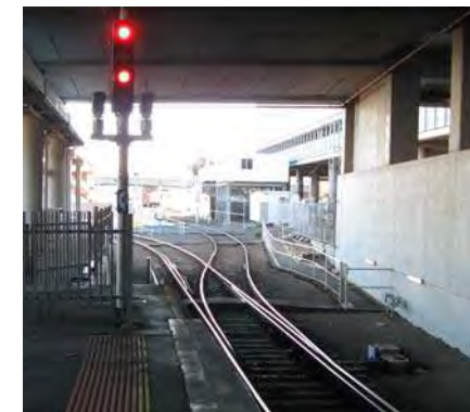
Turnout: (b.g+ s.g) Main to b.g Branch. 2 moving blades [Integrated 3rd rail transition]
