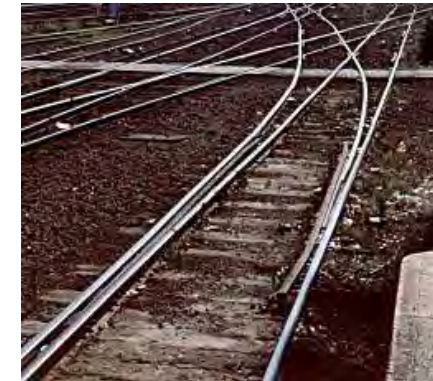
Divergence: (b.g+s.g) to s.g.Main & b.g. Branch. no moving blade
