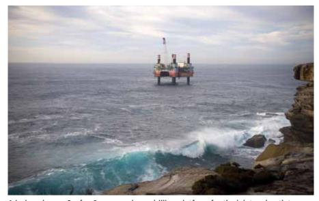
A jack-up barge, Seafox 6, was used as a drilling platform for the inlet and outlet shafts for the desalination plant. Construction of the plant was completed on time and under budget.
