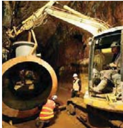
Installing pipes in the enlarged pumping station cavern
