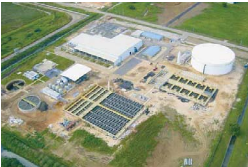
The Ionics Desalcott designed, owned and operated desalination facility at Point Lisas, Trinidad
