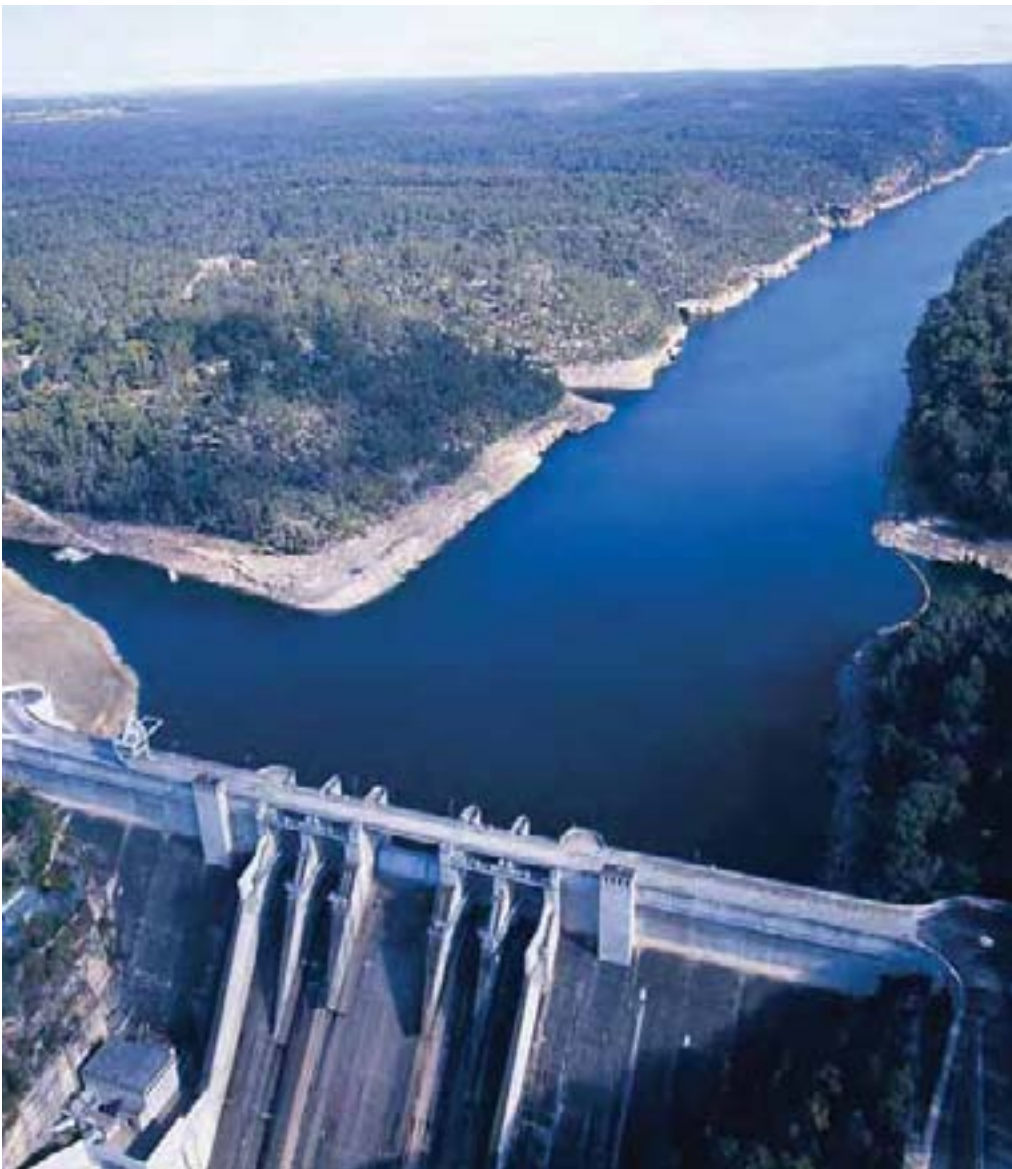
Looking upstream from Warragamba Dam
