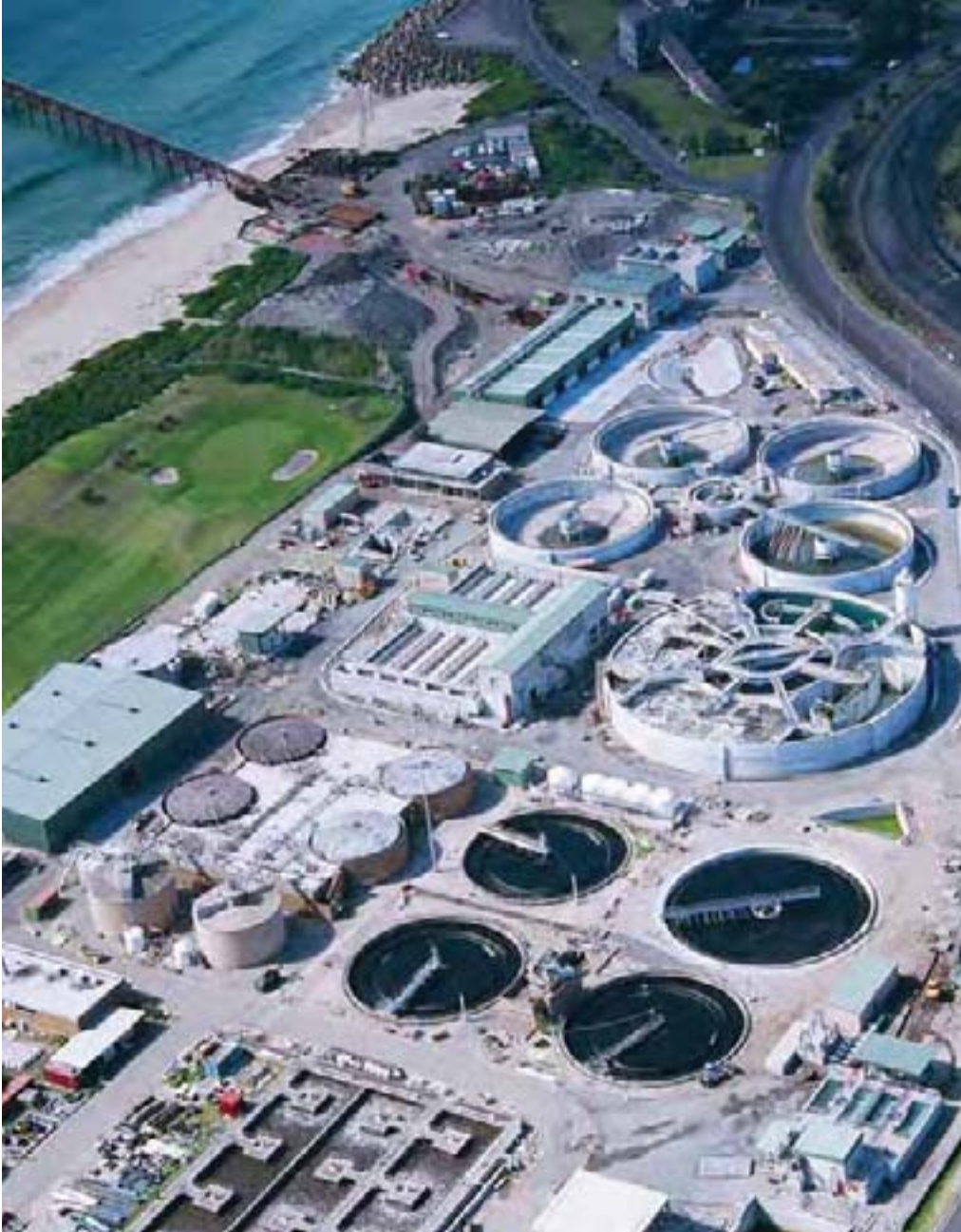
Wollongong Sewage Treatment Plant containing a recycled water plant.
