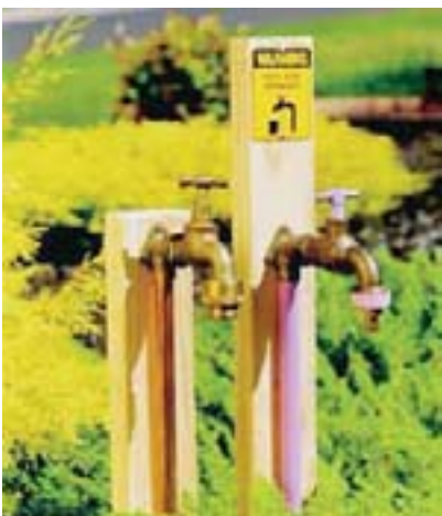
Purple recycled water and drinking water mains supply taps that are part of a typical dual reticulation scheme
