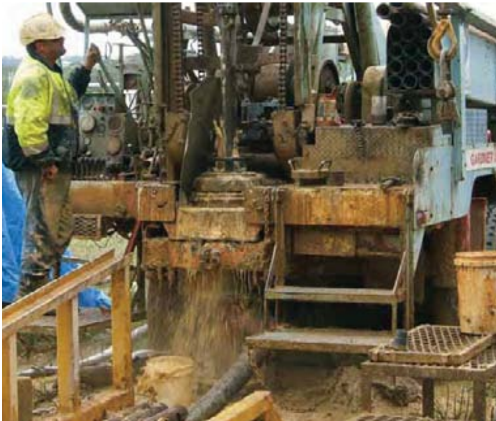
Groundwater bore drilling
