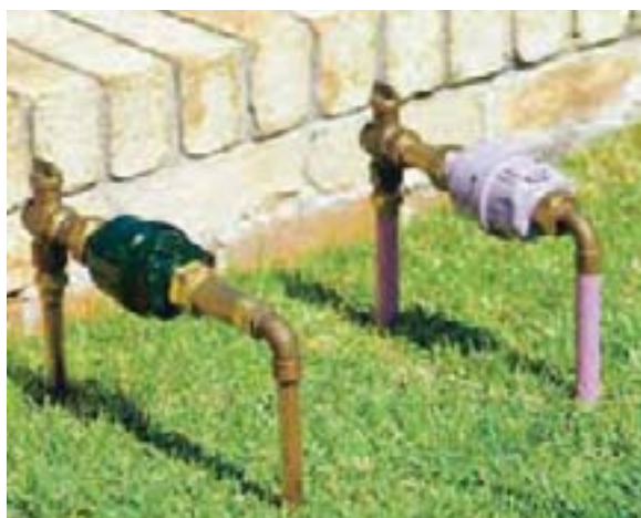
Purple recycled water and drinking water mains supply taps that are part of a typical dual reticulation scheme
