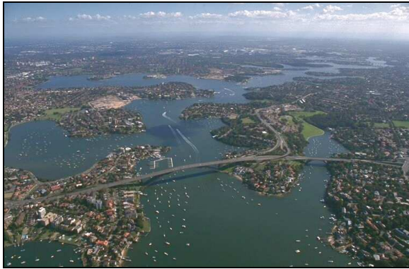
Parramatta River Estuary – Gladesville Bridge (DECC, 2008)
