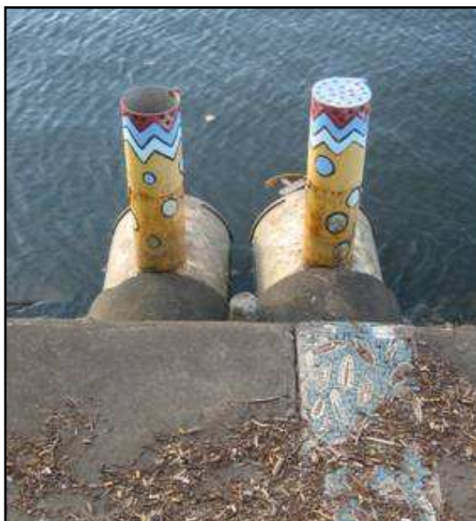
Stormwater Outlets into Iron Cove (4/3/2008)
