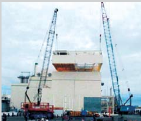
Construction of Koroit Milk Powder Building, Victoria
