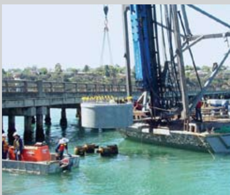
Construction of Sorell Causeway Bridge in Tasmania
