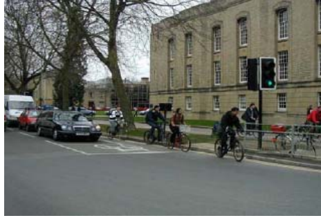
Advance stop lines (head start boxes) at a traffic signal intersection
