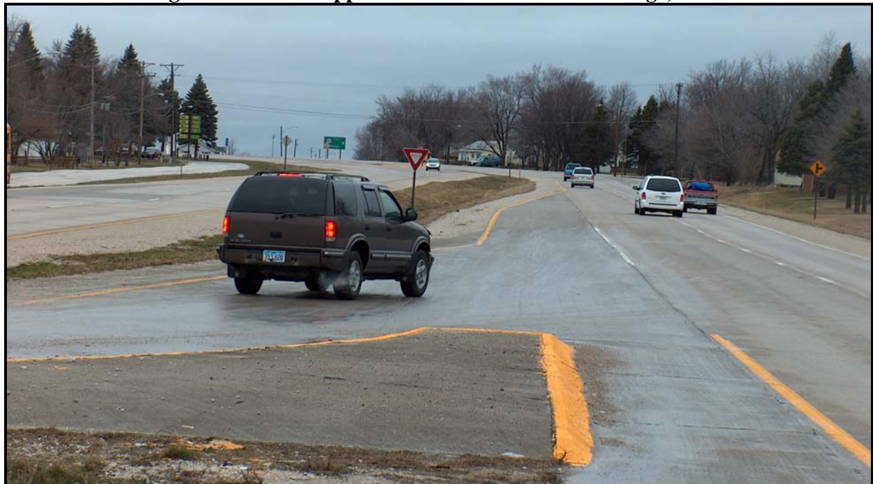
Figure 5 Looking North From South T-Intersection in Fort Dodge, IA
