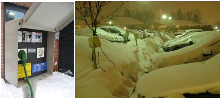
Fig. 17.2 Block heater poles typically have 2-hour timers; the starting time is selected by the user, and the heating time is fixed for 2 hours from the start. Lock Heater Pole (left) and View from the Car Parking Area of a Row House Condominium (right).
