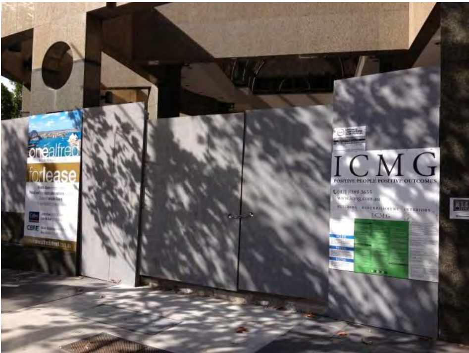
Figure 4-11: Temporary George Street Driveway at Goldfields House
