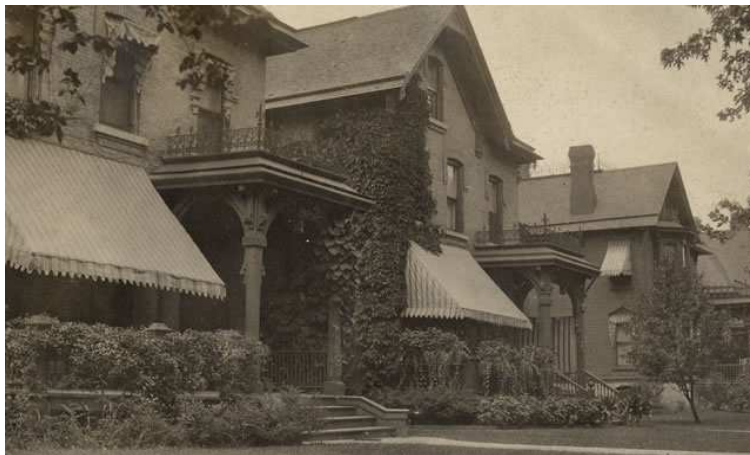
1903 North Cambridge Avenue, awning on the right
